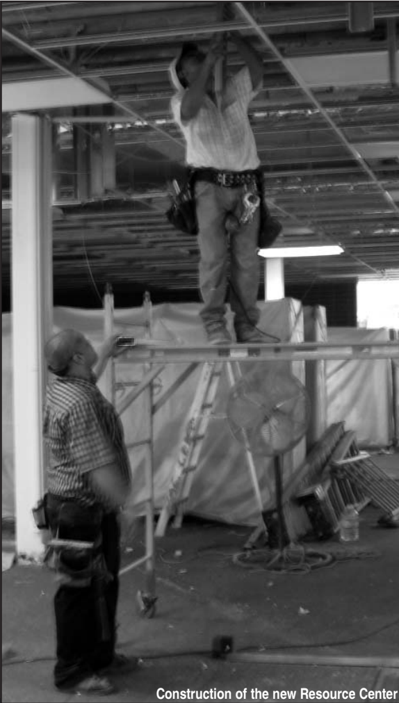
Construction of the new Resource Center
